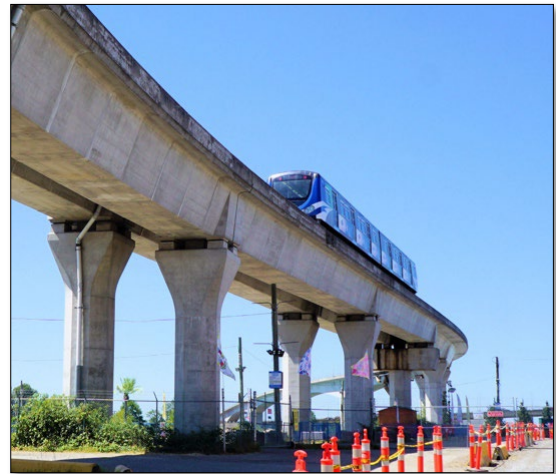
Figure 13. England, David. (Photographer). (2023). Canada Line Transit Bridge over middle arm to Sea Island. [Photograph].
