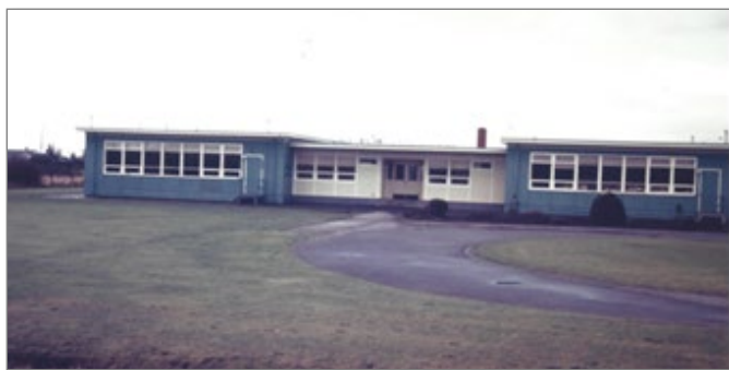
Duncan McDonald School, November 1962. City of Richmond Archives.
